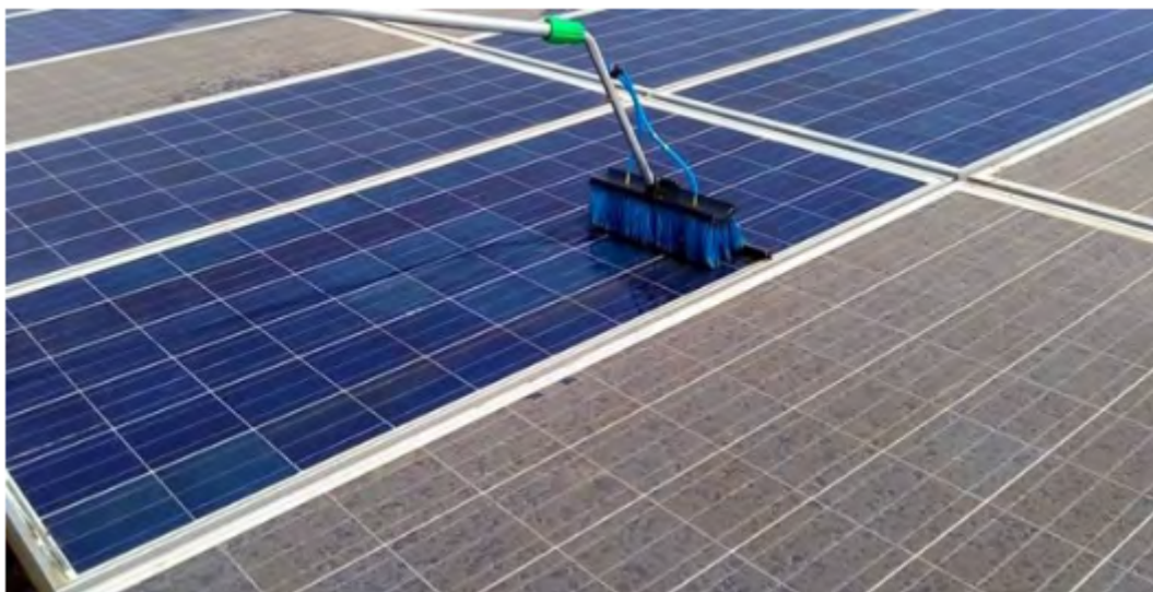
Fig. 1 Dust accumulation on panel surface Source: (Walz et al., 2018)
