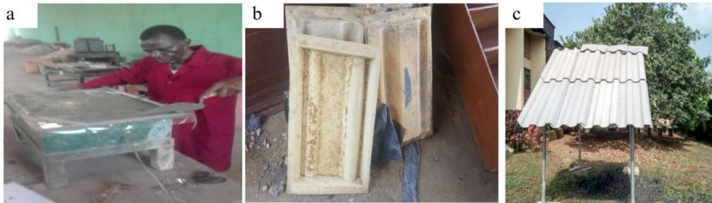
Fig 5: (a) Placing the mix on the Vibrating Machine (b) Mador Tiles as Produced (c) Application of the Mador Tiles
