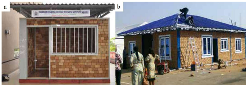
Fig7: (a) NBRRI Dismantlable One-Bedroom (b) NBRRI Dismantleable Three-Bedrooms
