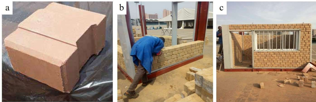
Fig 2: Compressed Stabilized Earth Block (a) the CSEB (b) Installation of the CSEB (c) Single Bedroom
